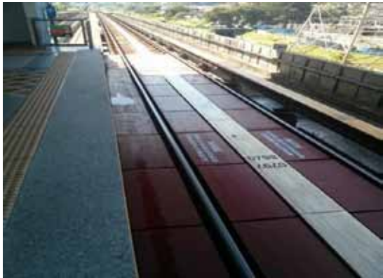
Sensor panels installed along rail tracks
